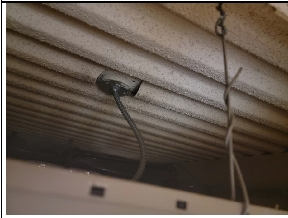
24. ACM HA 6 – Ceiling Texture on Metal Decking above Ceiling Tiles
