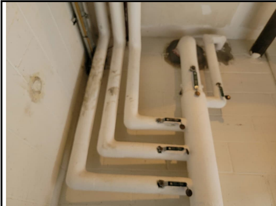
15. Fiberglass Pipe Insulation
