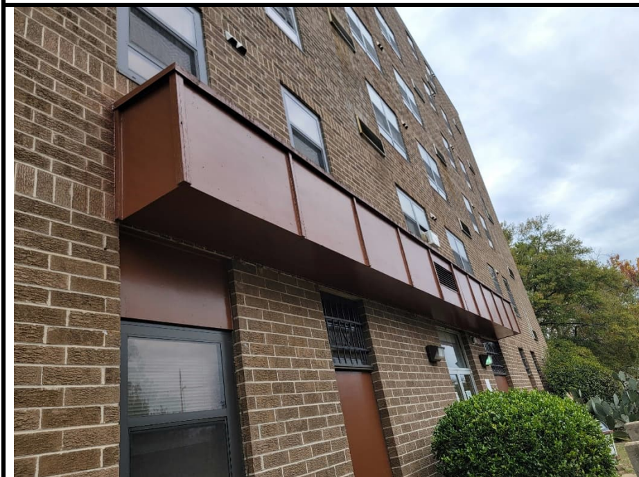
36. Assumed ACM Transite Panels on Exterior
