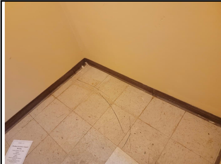
27. Assumed ACM 12"x12" Vinyl Floor Tile and Assumed ACM 4" Cove Base
